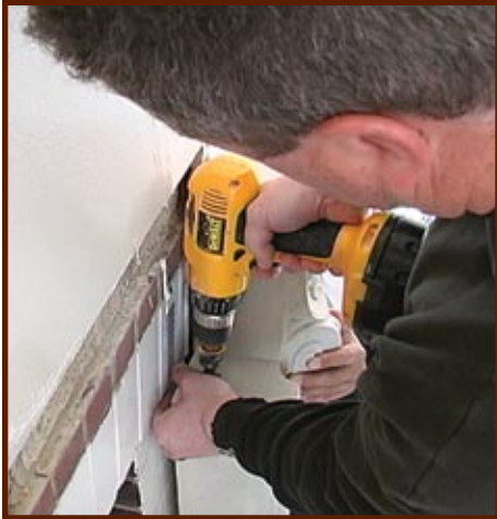
Above, the mason drills a pilot hole to anchor leg to wall.
