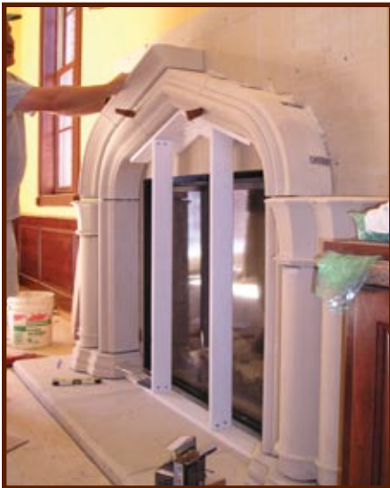
As shown above, the arch of this fireplace is externally supported until the mortar can set fully in place and final point up is done.
