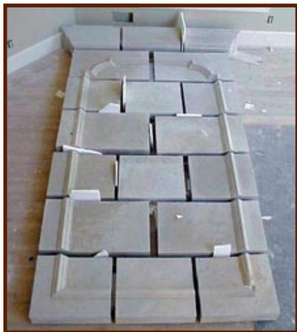
Before starting, layout the stone to dry and verify each piece. Scaffolding may be necessary to work on the upper portions of some mantels.
